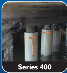
Timber Pile Structural Repair
