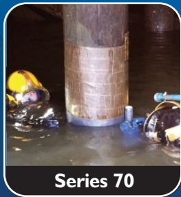
Timber Pile Protection
