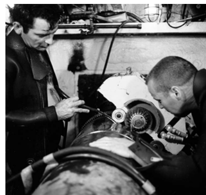
Ocean Systems divers monitoring the hydraulic pipe cutter (Christopher Swann)
