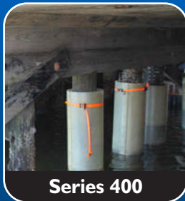
Timber Pile Structural Repair
