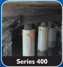
Timber Pile Structural Repair
