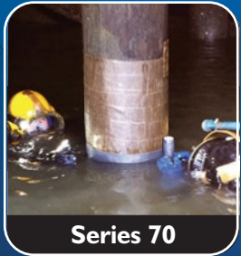
Timber Pile Protection
